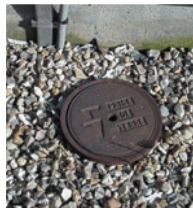
^ Lightning conductor earthing electrode
