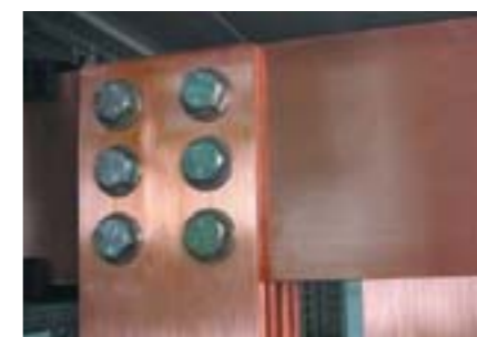
^ Connection on 120 x 10 bars (4000 A)
