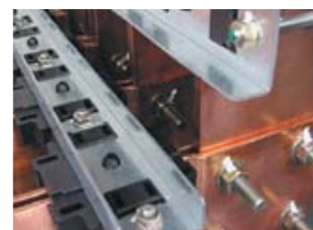
^ Connection on 120 x 10 bars (4000 A)
