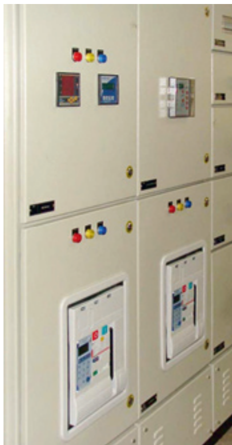
< Assembly with DMX 3 supply inverter
