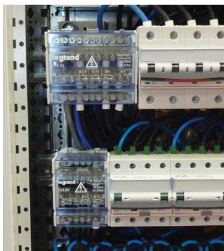
One-piece modular distribution blocks.
