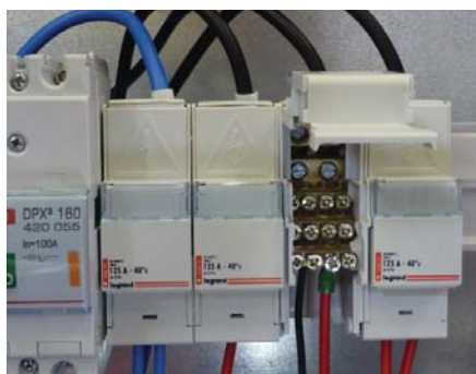
Single pole modular distribution block.
